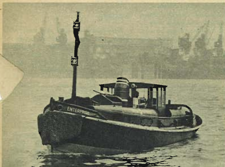
Powered by the largest British air-cooled diesel in Britain, this tug is operated by British Waterways in the Regent Canal Docks. The 96 h.p. Petteer propulsion unit gives an average speed of 9 knots and a static pull of 26 cwt.
